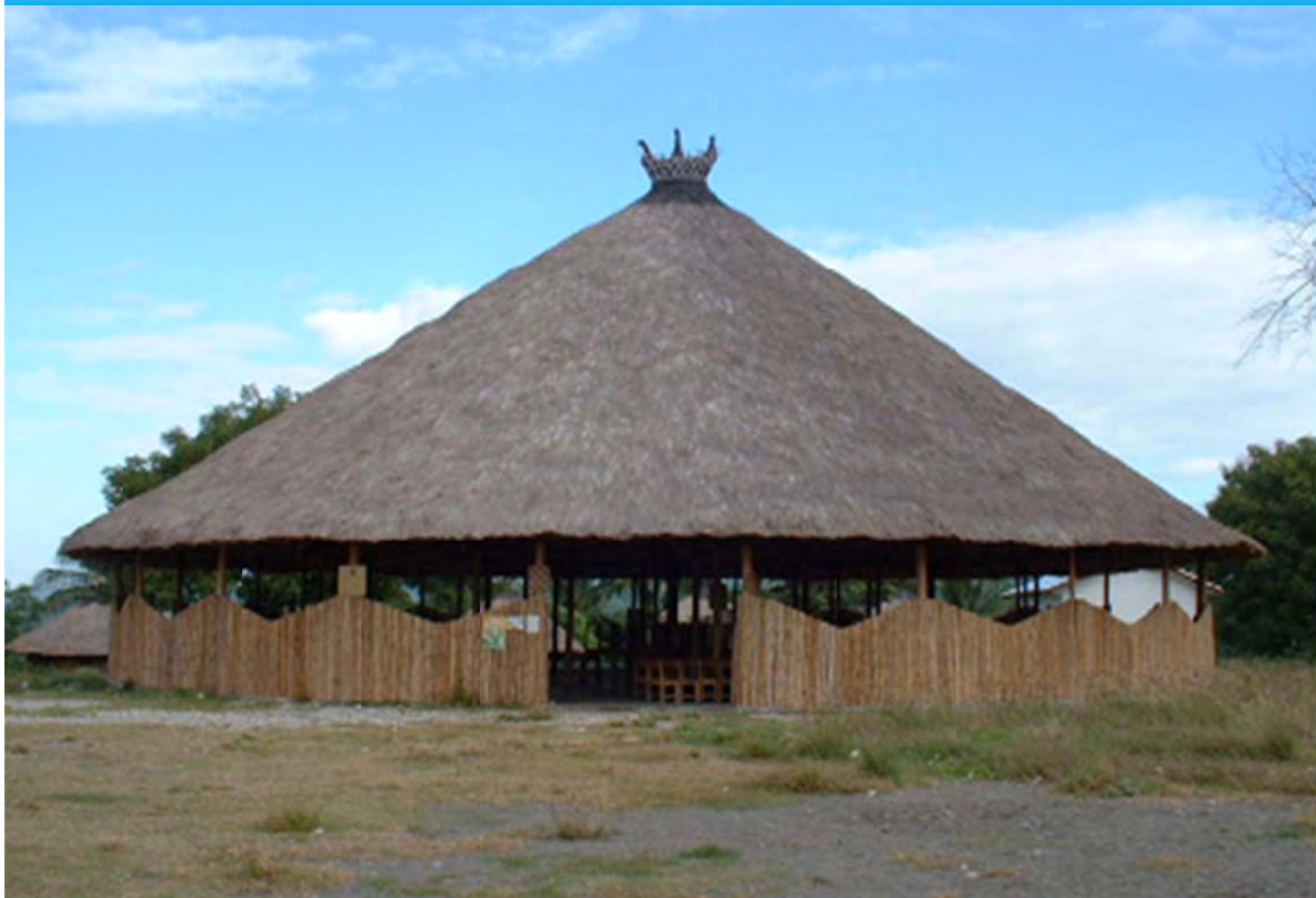
Community Centre in Covalima District Sentru Komunitade iha Distritu Covalima
